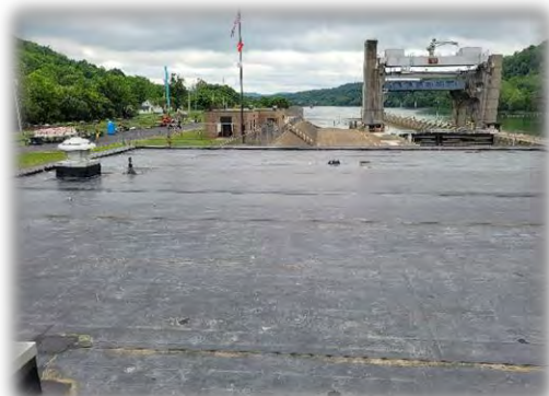
GRAY'S LANDING LOCK & DAM ROOF REPLACEMENT
